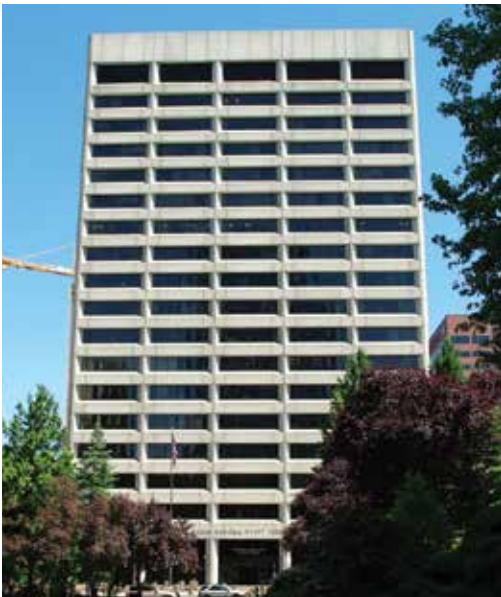
Prior to renovation.
